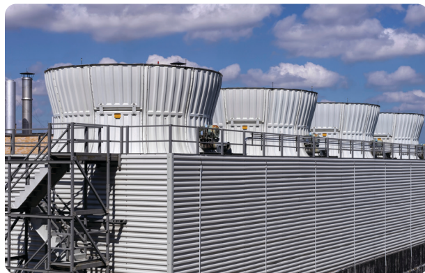
Heat is removed from Purdom's cooling water, producing steam.
