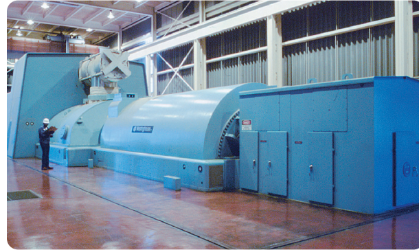
Hopkins' combined-cycle system powers two generators using the same amount of fuel as one.
