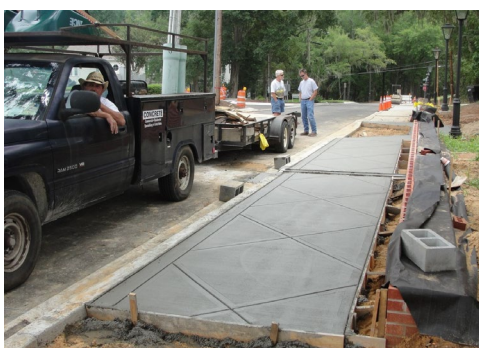
5th Avenue Sidewalk Construction
