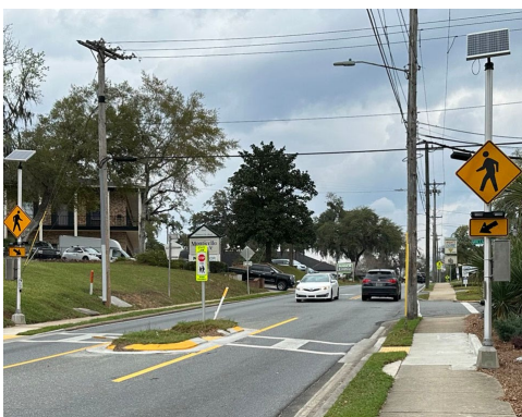
Pedestrian Crossing with RFB
