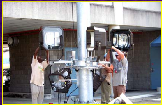
Apron Lighting Upgrade
