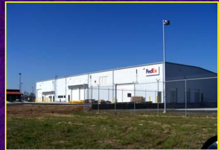
New FedEx Facility
