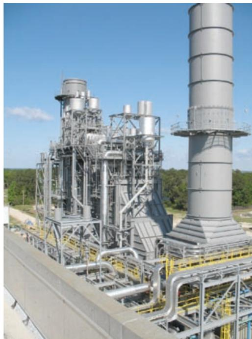
**1. Downstream of the gas turbine** is the bypass stack and the heat-recovery steam generator for the repowered Hopkins Unit 2
