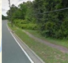
Existing Substandard Sidewalk
