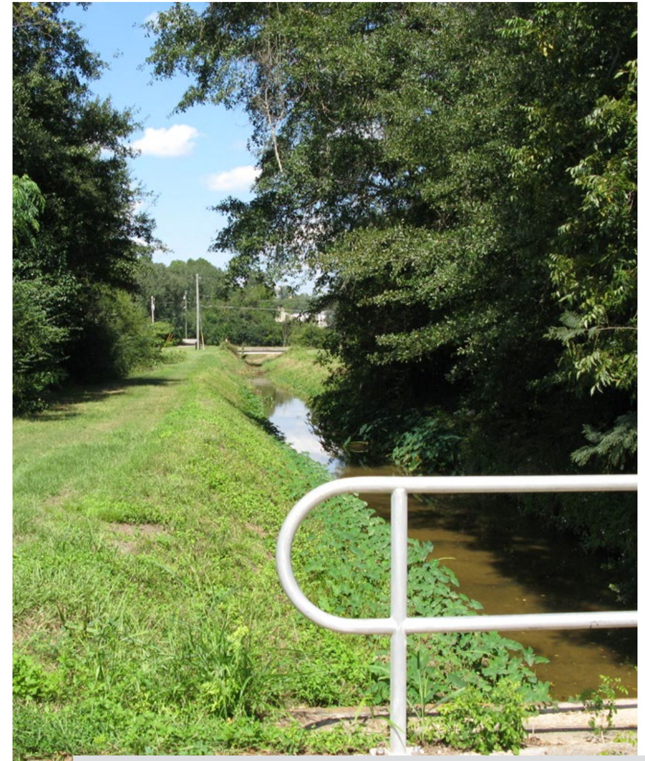
Drainage Channel near Tharpe Street
