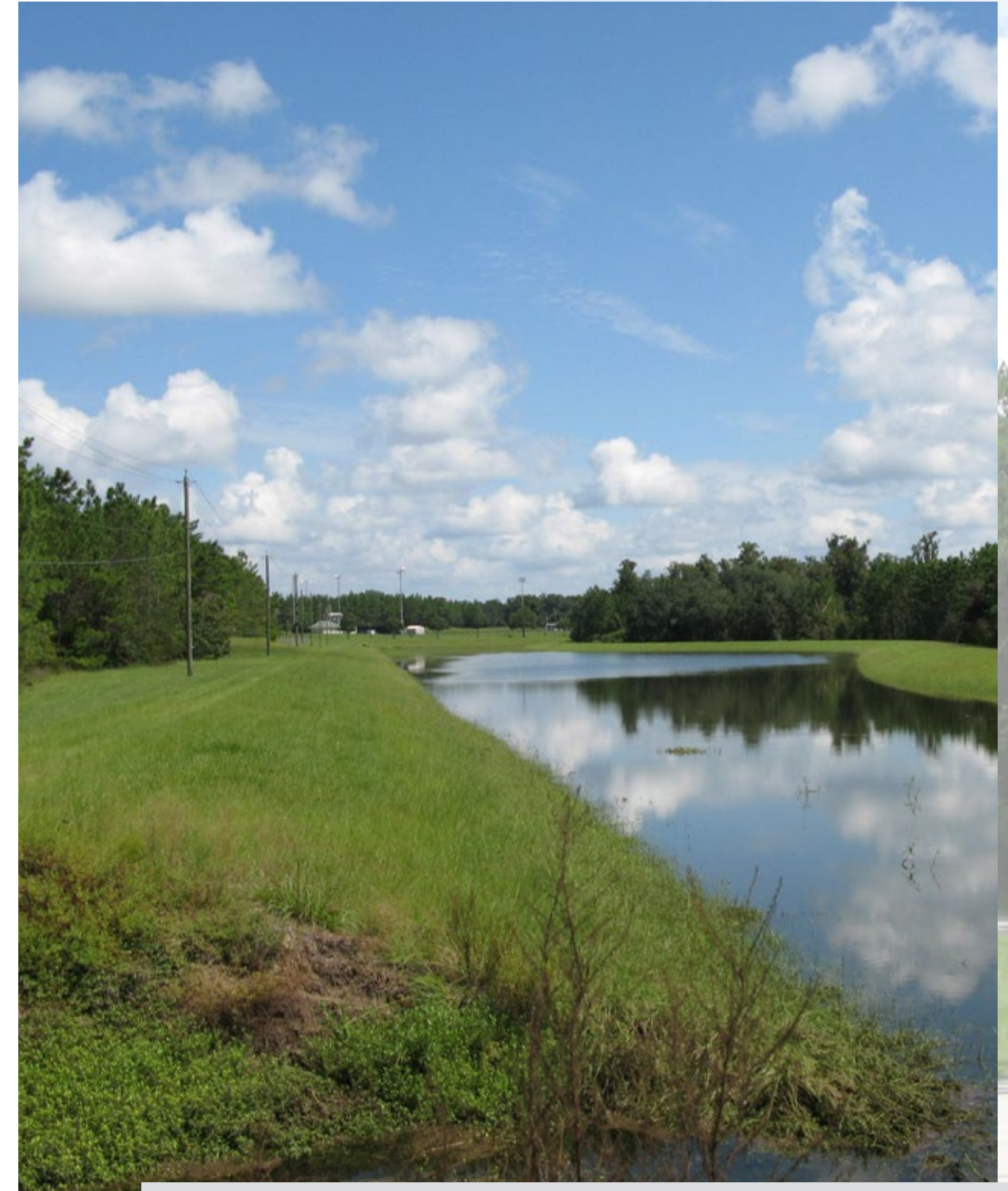
Stormwater Facility at Southwood
